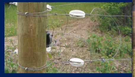
**Connect wires in parallel at the end of runs.** A good way to increase the ability of a fence to carry voltage is to connect all the wires at the beginning and end of runs of multi-wire fence. This allows the multiple strands of high tensile wire to function as one large wire that can carry higher levels of voltage.
